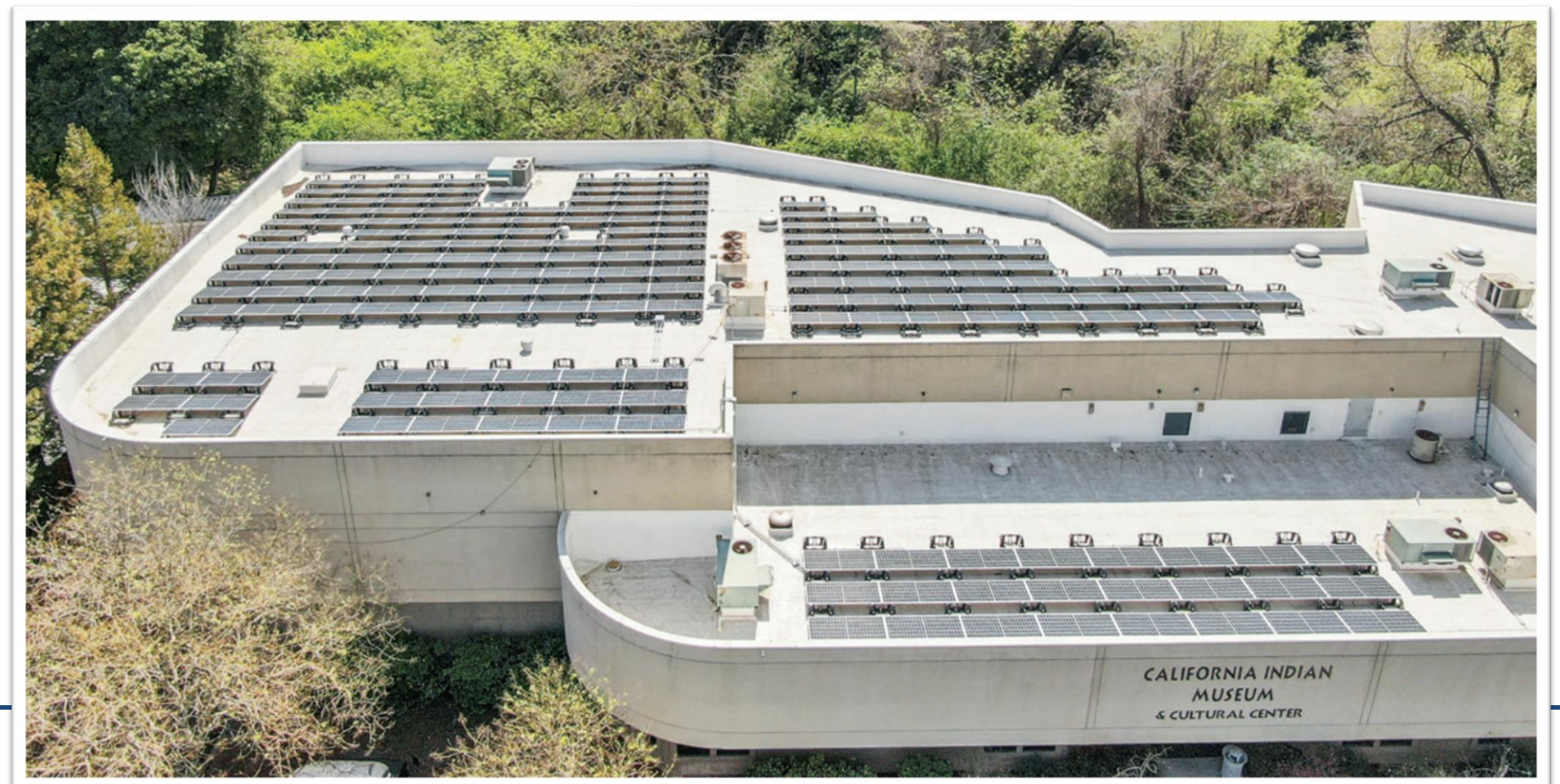
Solar array at California Indian Museum and Cultural Center. CIMCC was a TAF awardee.
