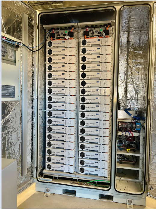
Open battery storage cabinet with cells visible.
