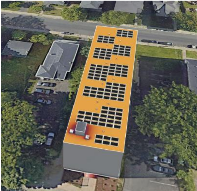
Figure 2: Representative design of a 46-kW rooftop solar system for the a mid-rise multifamily apartment building.
