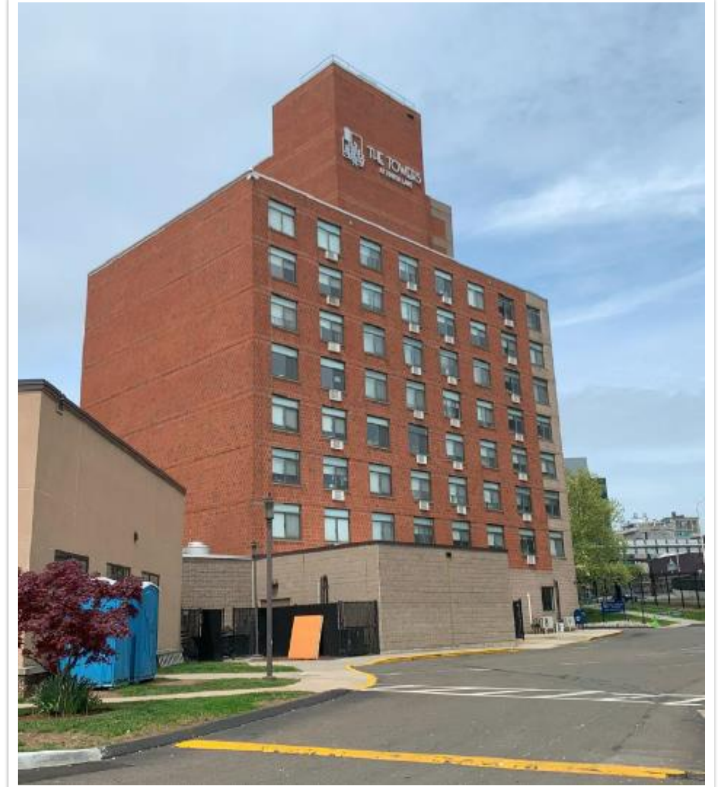
The Towers at Tower Lane Credit: AMS
