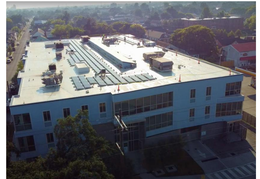
Solar array installed at CrescentCare health clinic in New Orleans, Louisiana. Credit: Together New Orleans.
